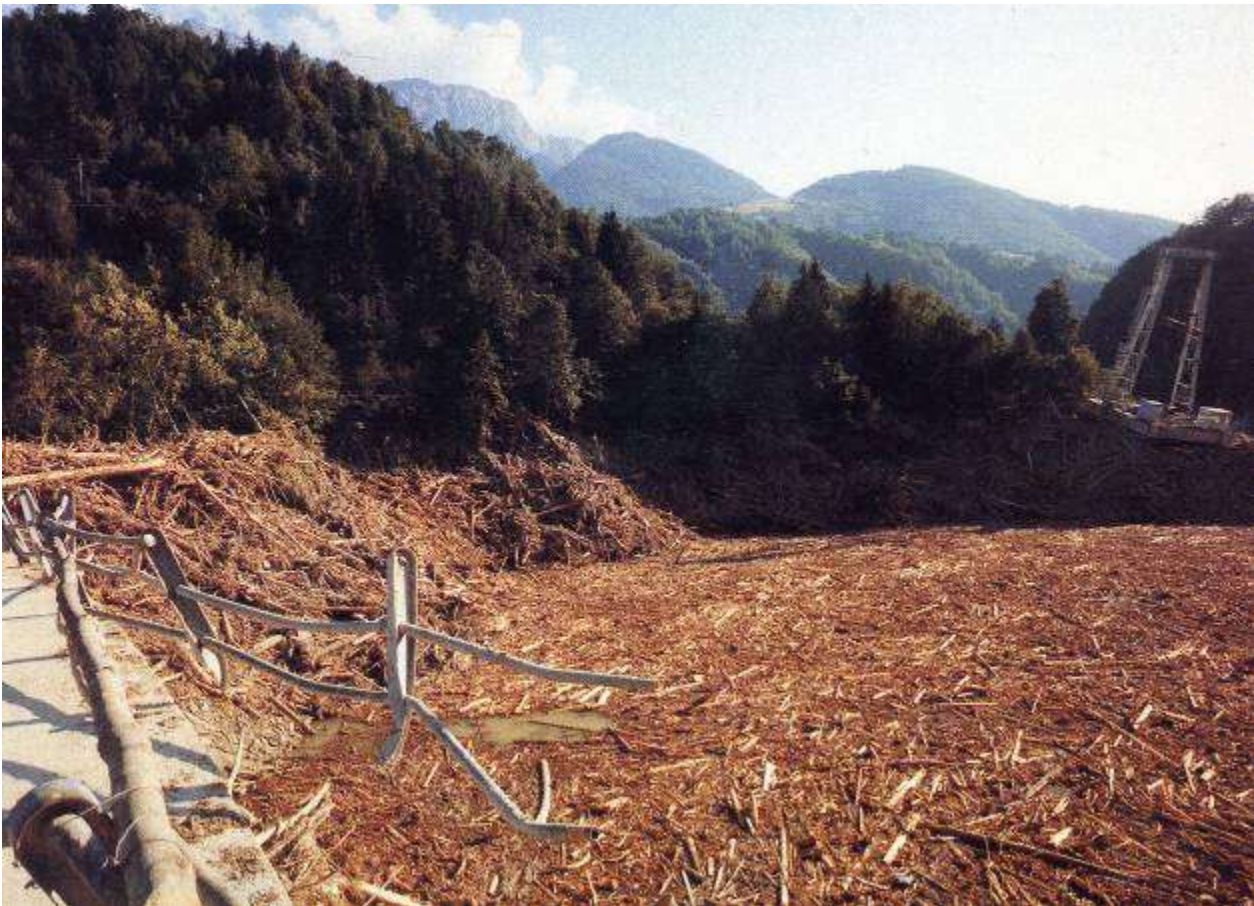
Figure 3-6: Debris in Palagnedra Dam , Switzerland following record floods
