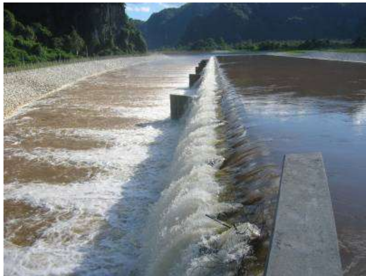
Figure 3 -4: On site view of the aeration in operations for 150 m 3 /s ( EDF)
