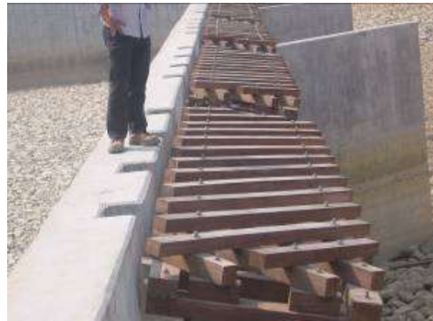
Figure 3 -3: View of the flows detail on the aeration weir model test for 150 m 3 /s (Hydraulic Laboratory of Constructions; University of Liège Belgium) and on site implementation
